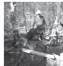
Clayton Smith and Tony Barrington build a bridge at Norton Preserve.
